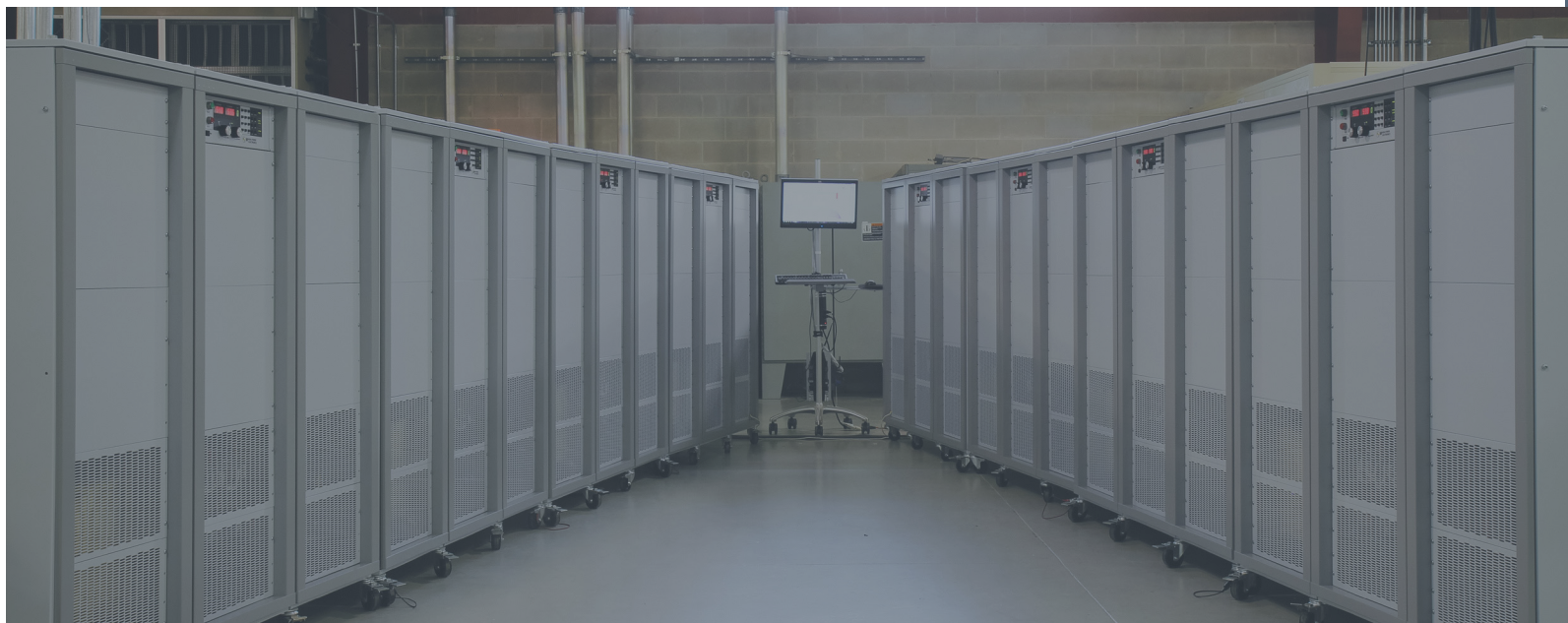
Qty (8) 250 kW MT Series units in master-slave parallel to form a 2 MW system
